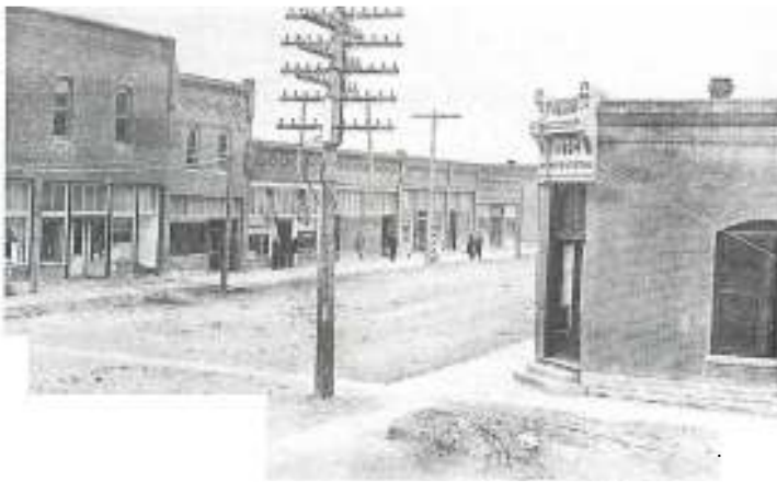
Clay Street, Bronson, KS-looking north from fire bell tower
