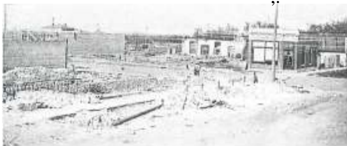
Rebuilding Bronson, KS 4-11-10
